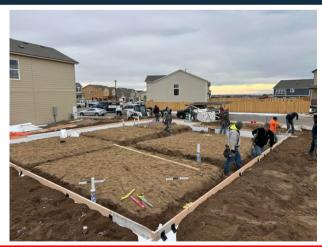
Did you know that the NEW Adjustable Form is superior to the Arctic Form? That's right! With the Adjustable Mono Slab® EZ Form provides over 51 inches of frost protection. The Adjustable Frost-Protected Shallow Foundation form Easy to level to +/- 1/2 inch The waste and garbage has been eliminated (no need to breakaway the top triangular portion) Complies with 2022 IRC, IBC, and IECC Codes.
